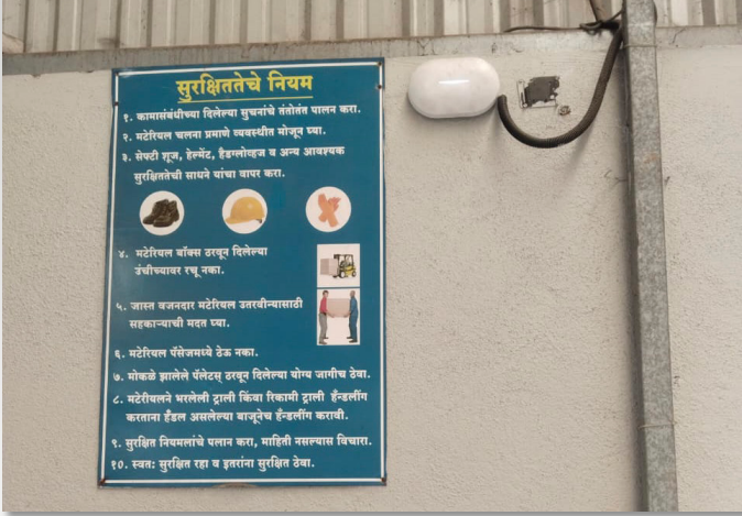
AP6 Mounted Inside the Warehouse
