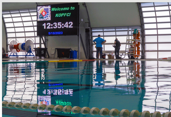
Installing an AP6-Pro at KOPFC
