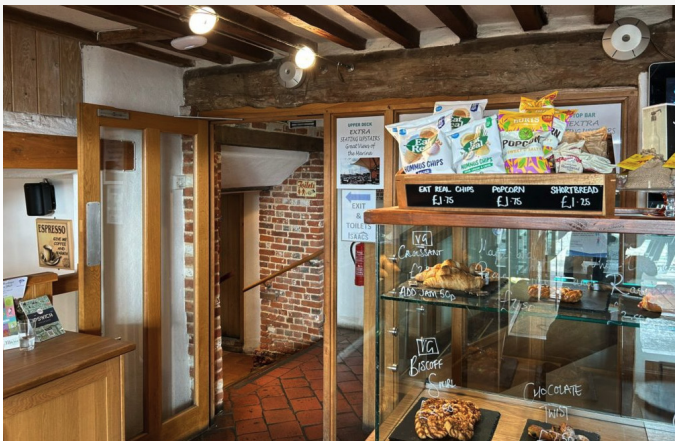
AP6-Pro Installed in the Coffee Tavern
