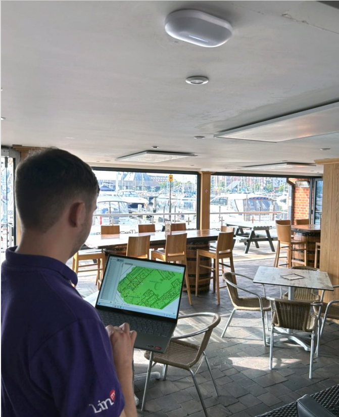
Scanning Environment After Installation of Alta Labs APs
