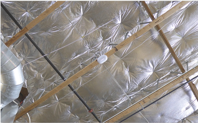
AP6-Pro Installed in the Fitness Culture Gym
