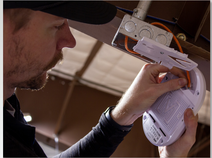
Installing the AP6-Pro at the Be More Sports Complex
